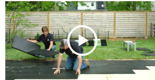
HOW TO INSTALL A GRANITE SLAB PAVER PATIO IN HALF THE TIME WITH EZ BASE
