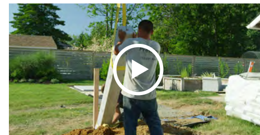
UPGRADE YOUR OUTDOOR LIGHTING: HOW TO INSTALL A GRANITE LAMP POST
